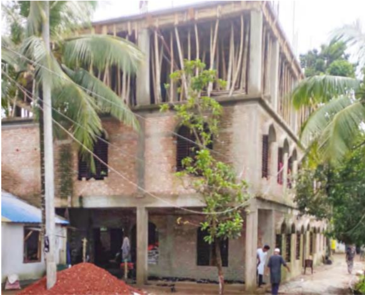
Fig: The three floors of the five-storey mosque under construction have been completed (2020).
